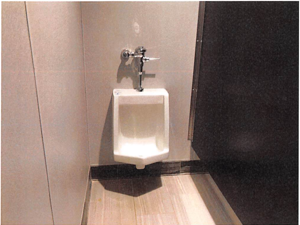
Figure 12 – Restroom Building -Mens
