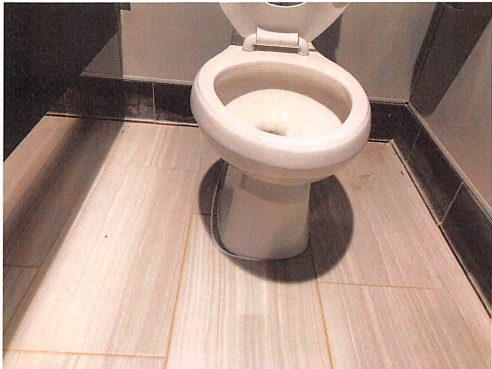
Figure 8 – Restroom Building - Womens
